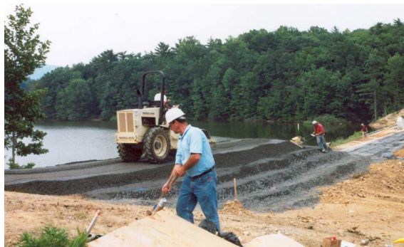
Fig. 4. Installation of Roller Compacted
