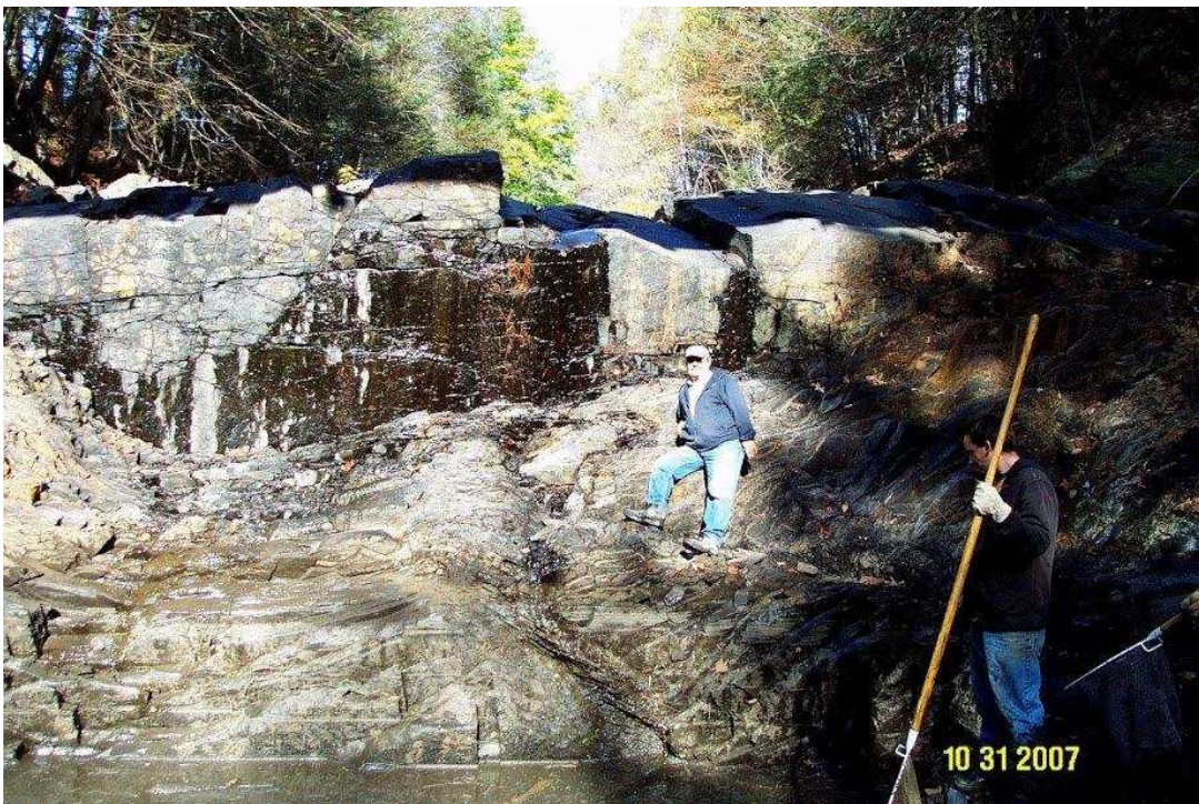
Fig. 7. The “dry” waterfall in 2007 when the outflow was closed showing the Montebello Sandstone Member
